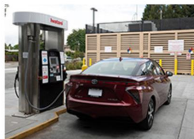
Iwatani Mountain View H2 Fueling
