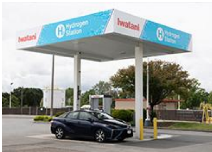
Iwatani West Sacramento H2 Fueling
