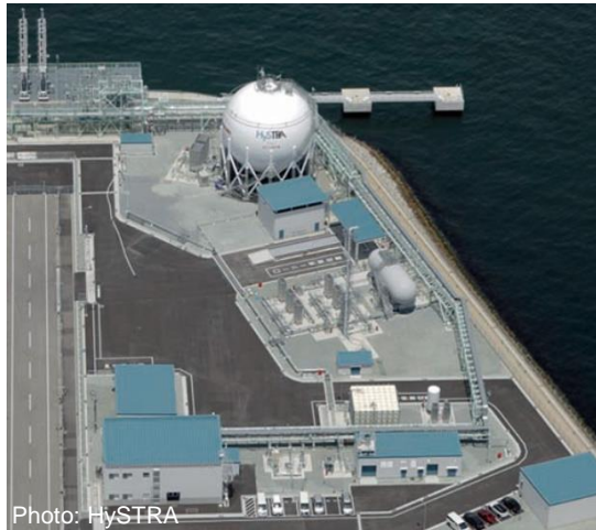
LH 2 receiving terminal
