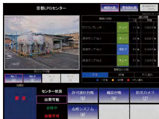
Checking damage by camera using the gas center security system
