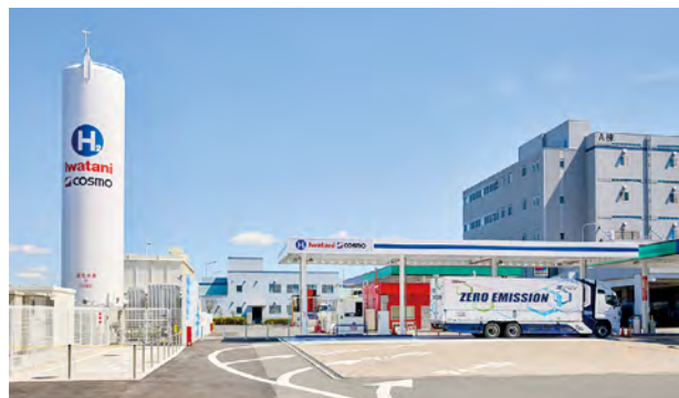
Iwatani Cosmo Hydrogen Refueling Station Heiwajima
