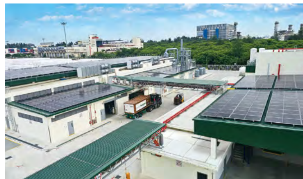
The new gas center on the island of Jurong, Singapore
