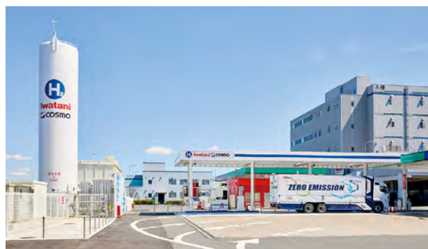
Iwatani Cosmo Hydrogen Refueling Station Heiwajima
