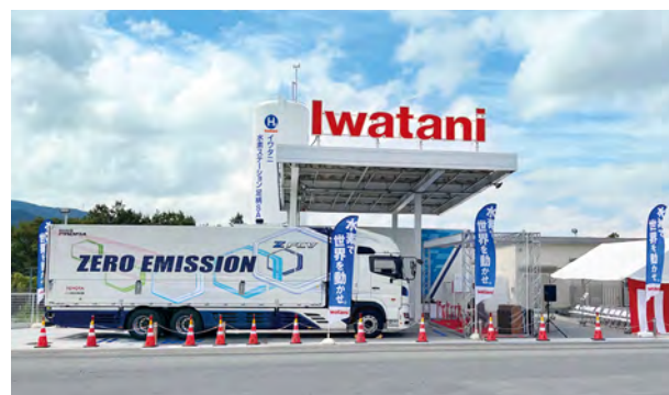
Iwatani Hydrogen Refueling Station Ashigara SA
