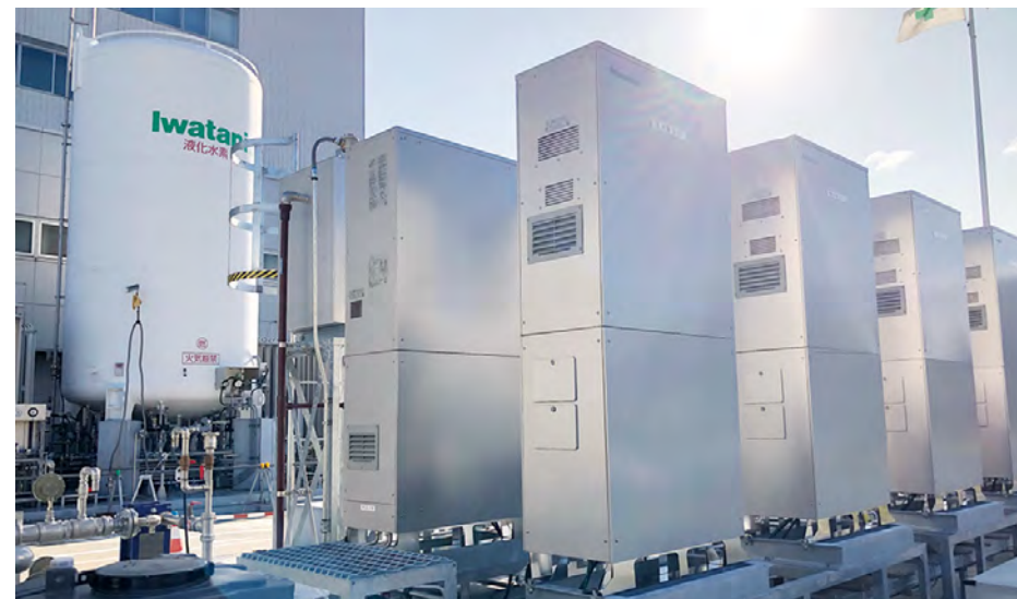
Pure hydrogen fuel cells (20 5 kW cells) adopted at the Iwatani R&amp;D Center
