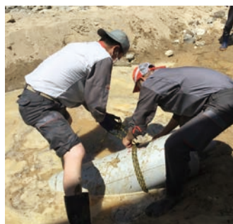
July 2018: Heavy rainfall in western Japan
