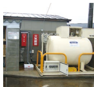
Disaster-ready LPG bulk storage tank
