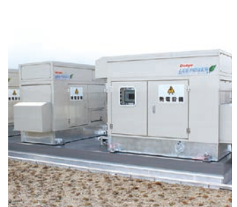
LPG power emergency generator
