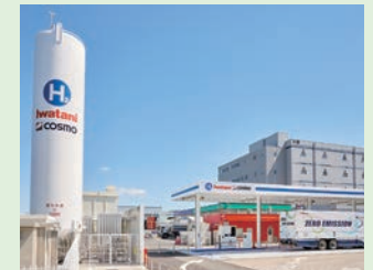
Iwatani Cosmo Hydrogen Refueling Station Heiwajima
