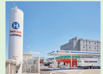
Iwatani Cosmo Hydrogen Refueling Station Heiwajima
