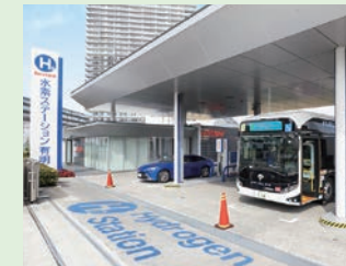
FC bus -adapted hydrogen-refueling station
