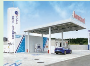
Hydrogen-refueling station equipment
