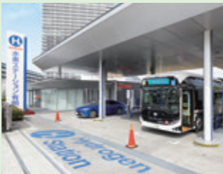
FC bus -adopted hydrogen-refueling station
