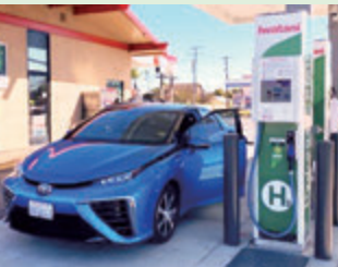
US hydrogen-refueling station
