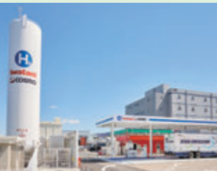
Iwatani Cosmo Hydrogen Refueling Station Heiwajima
