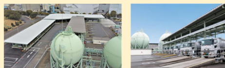
Negishi Liquefied Gas Terminal
