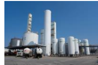
Air separation plant (Jiaxing, China)
