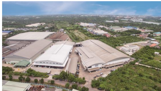
portable cooking stove plant in Thailand
