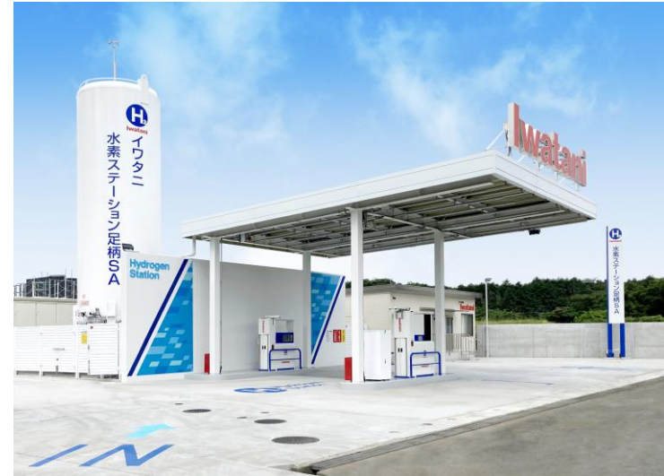
Iwatani Hydrogen Refueling Station in Ashigara SA
