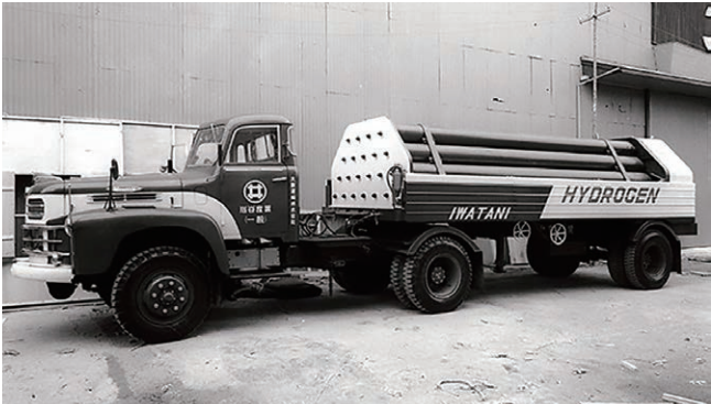
A hydrogen trailer, developed in 1960
