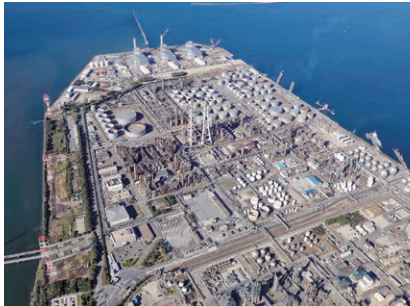
Chiba Refinery of Cosmo Oil Co., Ltd.
