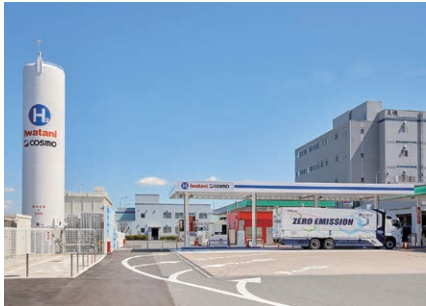
Iwatani Cosmo Hydrogen Refueling Station Heiwajima
