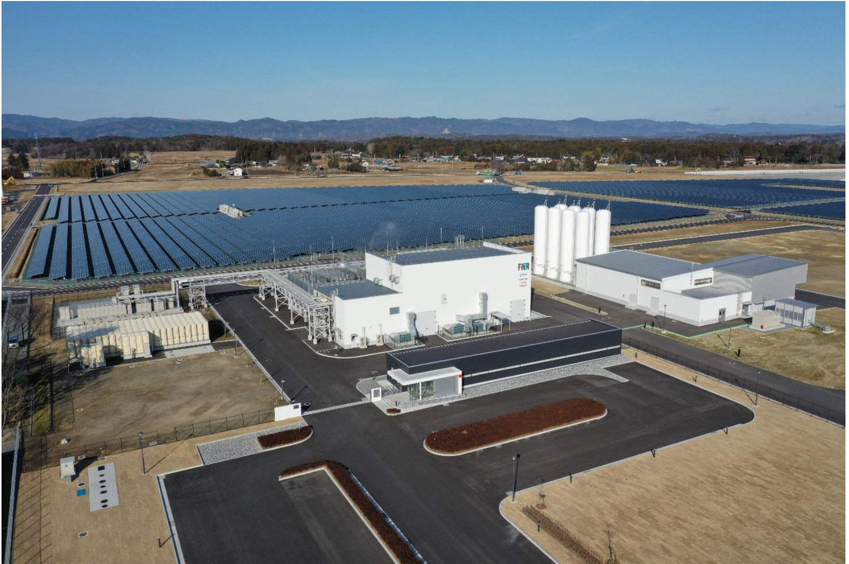
Fukushima Hydrogen Energy Research Field completed construction
