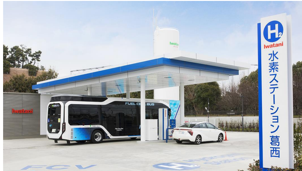
Iwatani hydrogen-refueling station in Tokyo Kasai
