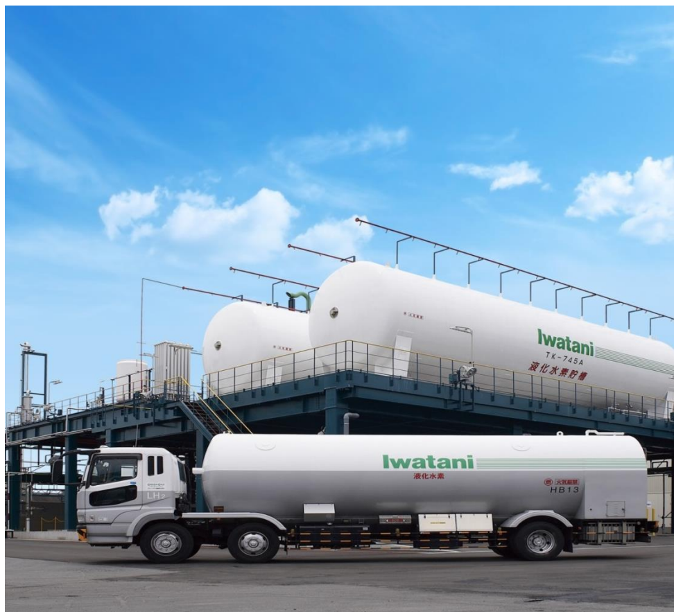
Yamaguchi Liquid Hydrogen Corporation
