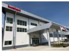
Portable gas cooking stove production plant
