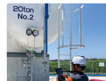
Plant facility inspection using tablets
