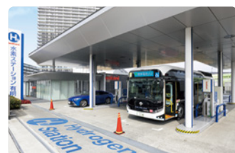
Hydrogen-refueling station for FC buses
