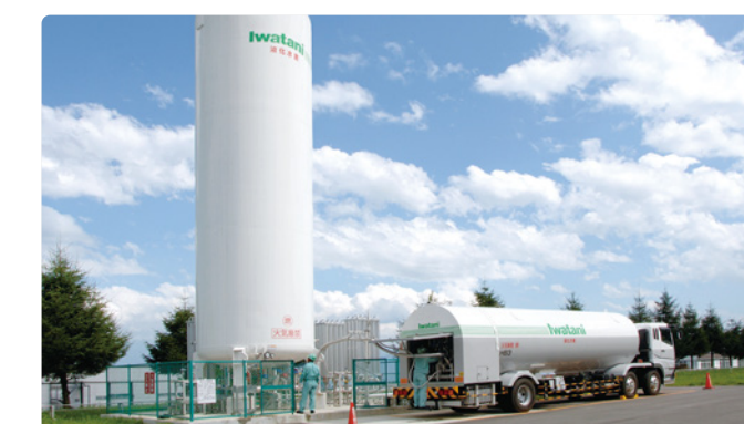
A tanker truck and storage tank, both essential to supplying liquid hydrogen
