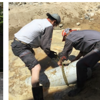
July 2018: Torrential downpours in western Japan
