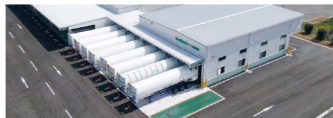
The Tokyo Helium Center, completed in April 2019
