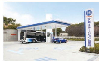
Iwatani Hydrogen Refueling Station in Tokyo Kasai can refuel FC buses.
