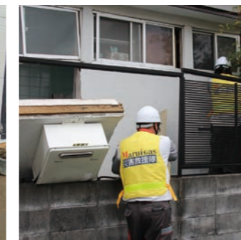
April 2016: Kumamoto Earthquake
