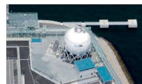
Aerial photograph of a liquid hydrogen loading terminal Photo courtesy of HySTRA
