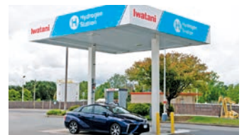
Hydrogen refueling station in the United States
