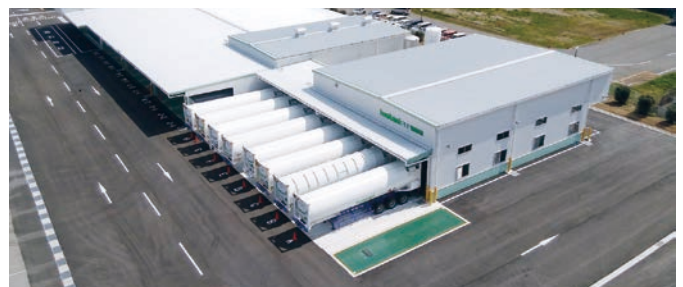
Tokyo Helium Center, completed in April 2019
