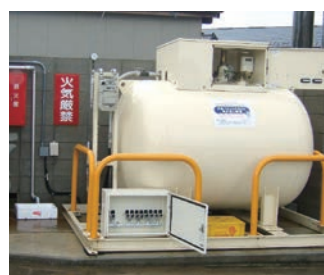
Disaster-ready LPG bulk storage tank
