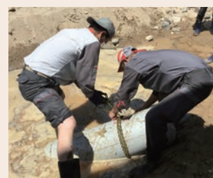
July 2018: Heavy rainfall in western Japan
