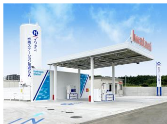
Iwatani Hydrogen Refueling Station in Ashigara SA
