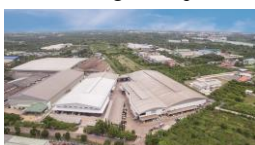
portable cooking stove plant in Thailand
