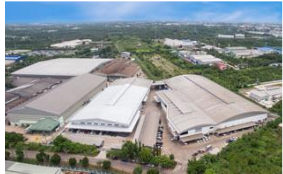
(Metal processing plant in Thailand)
