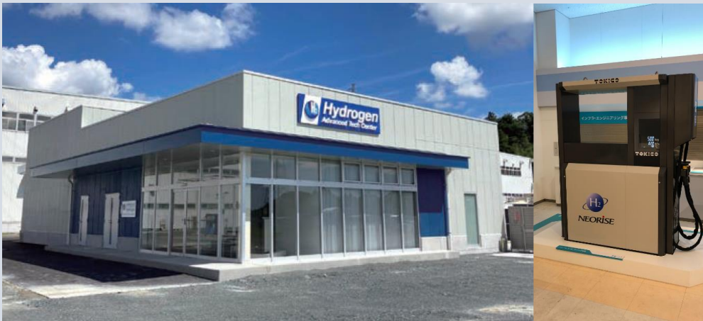
Technology Development Center (Operation is started from September 1, 2022) H2 dispensers
