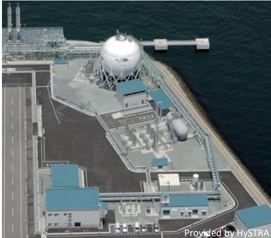
Liquefied hydrogen loading terminal (Japan)
