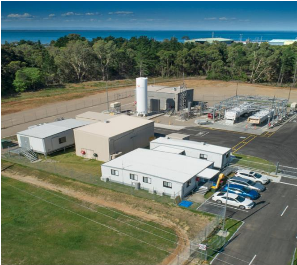
Hydrogen liquefaction and loading terminal (Australia)
