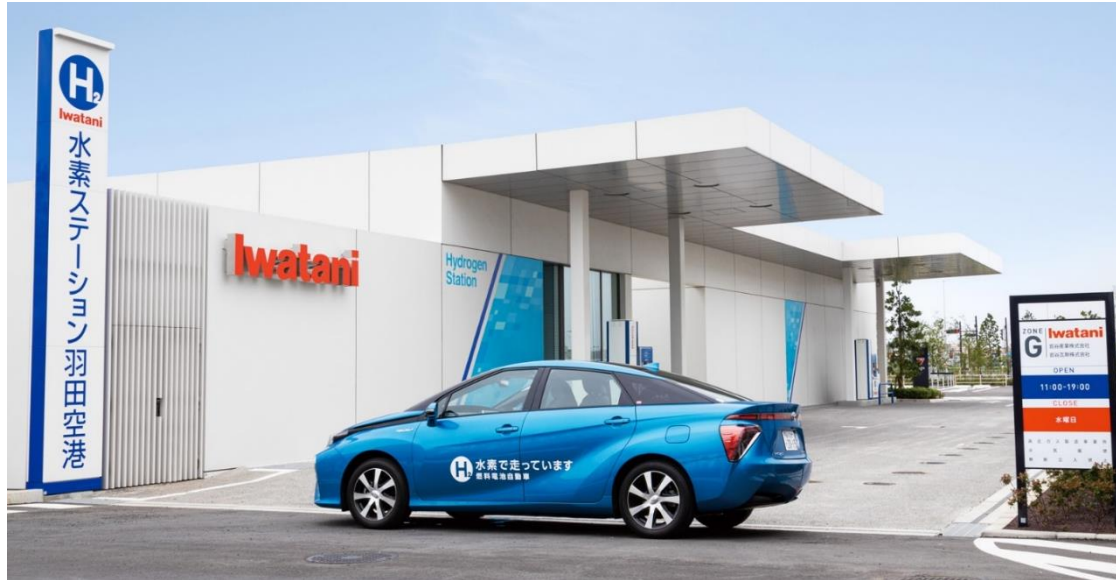
Iwatani hydrogen-refueling station in Haneda Airport
