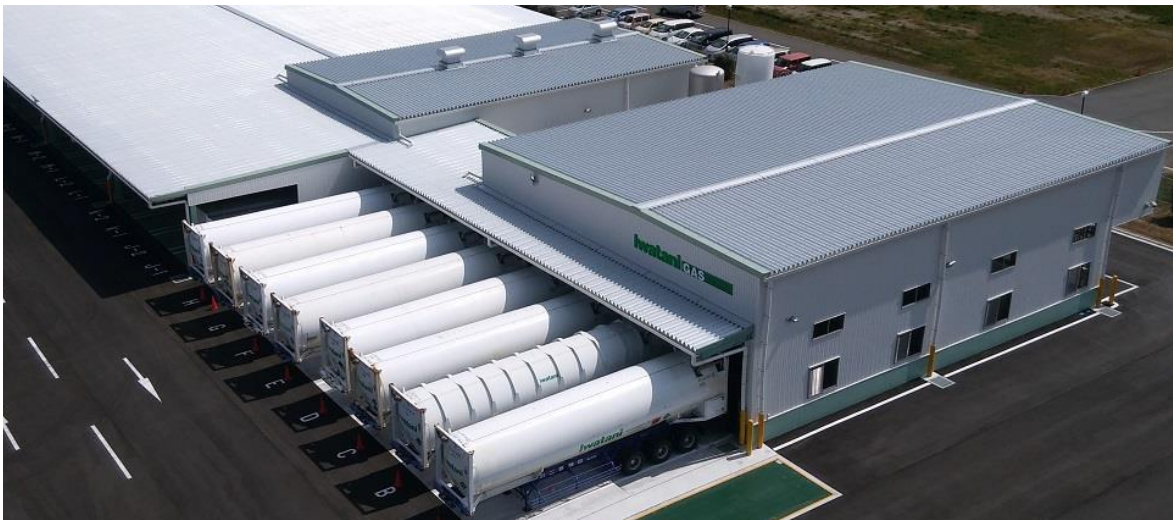
Tokyo-helium center (new construction)
